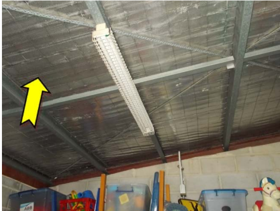
Photo 1. Interior, roof space, insulation – suspected SMF sarking insulation.
